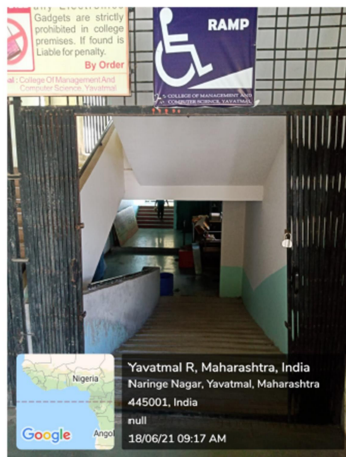
Ramp for Disable Person to Access Library, Computer Lab & Electronics Labs
