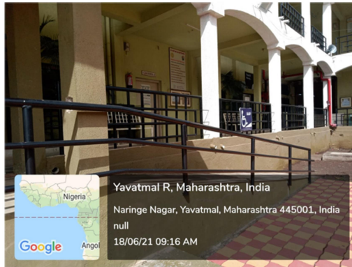
Ramp for Disable Person to Access Class rooms and admin office
