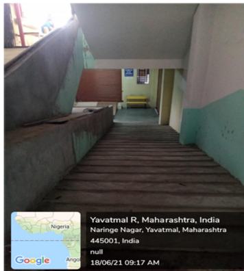
Ramp for Disable Person to Access Library, Computer Lab & Electronics Labs
