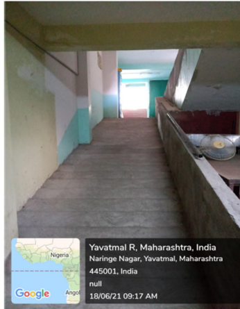
Ramp for Disable Person to Access Library, Computer Lab & Electronics Labs
