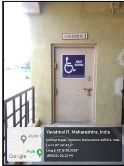
Rest Room With facilities
