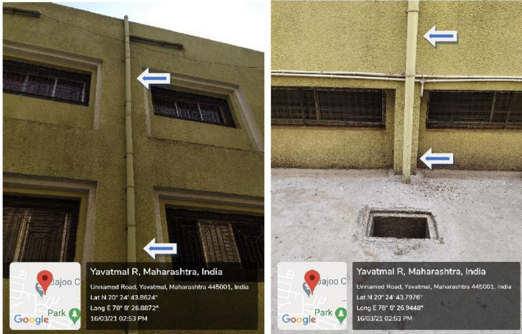
Pipeline of Water Harvesting System
