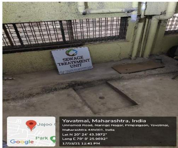
Sewage Treatment Plant in college
